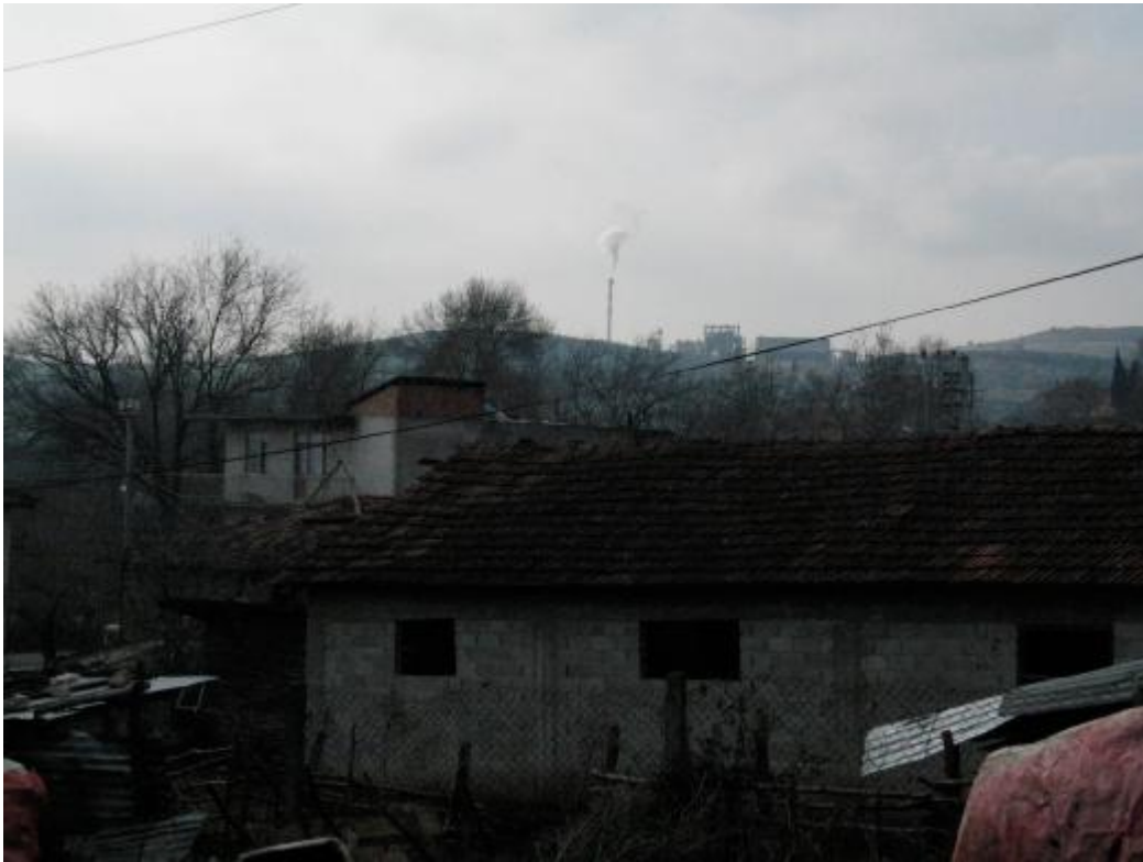
Photo 1: View at the incinerator from sampling place. Photo by: Greenpeace & Bumerang.
