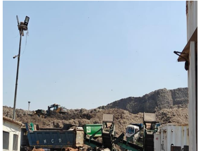
Figure 7: Okhla landfill site
