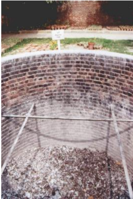
Pictures 9 - 11: Waste incineration residue in the deep hole - storage built in the area of hospital. Cover of similar hole in another hospital. Double chamber kiln in one of Pakistani medical waste incinerators. Photos by: Jindrich Petrlik
