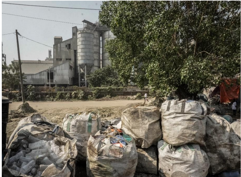
Plastic wastes are stored in front of cement industry. Source: ESDO, 2022
