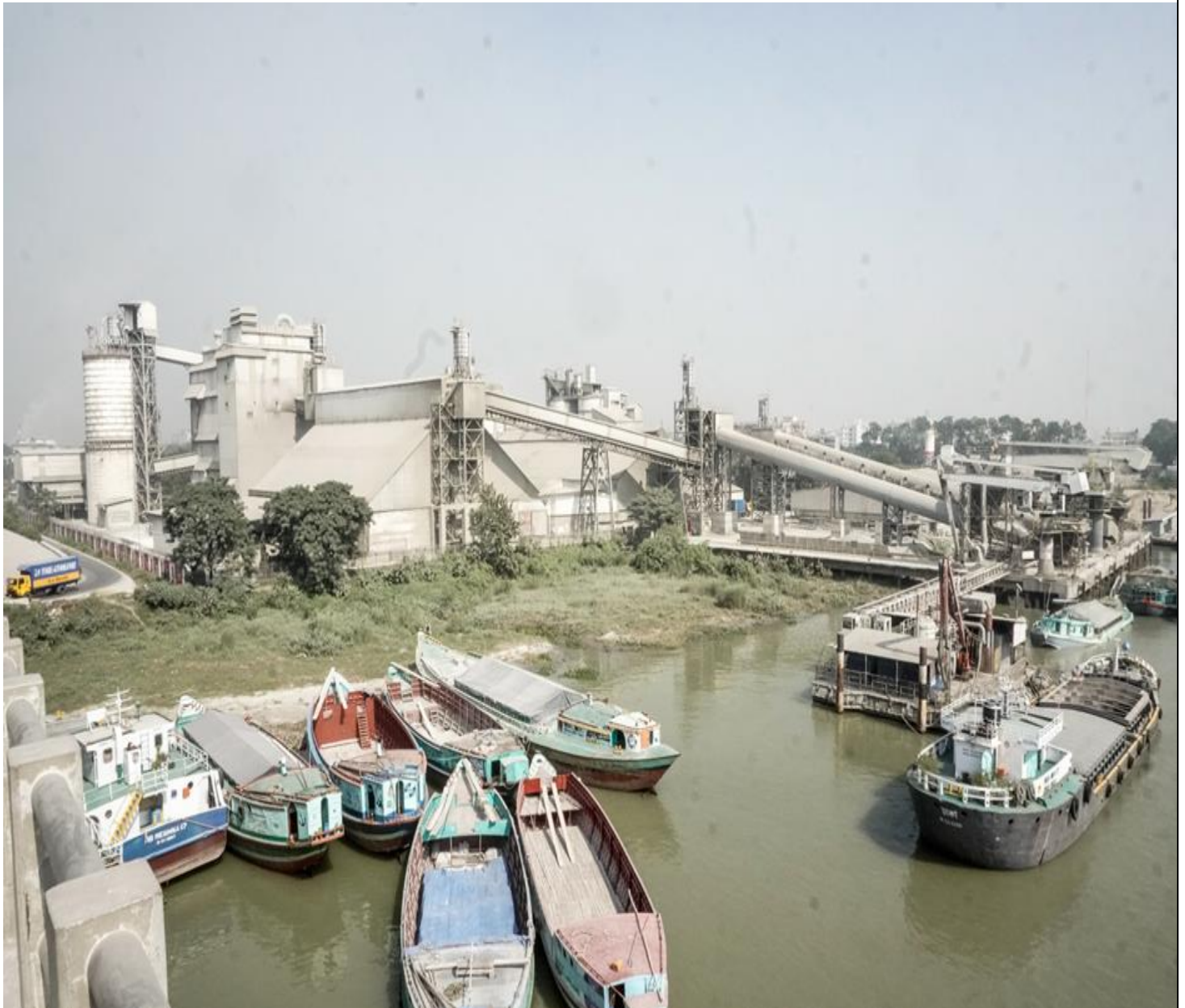
Figure 1: The Fresh Cement factory has many boats for transporting raw materials (cement producing stones and fuels like coals, woods, plastics, tyres and so on) or finished products. Here are some boats that are waiting for cement uploads. Source: ESDO, 2022
