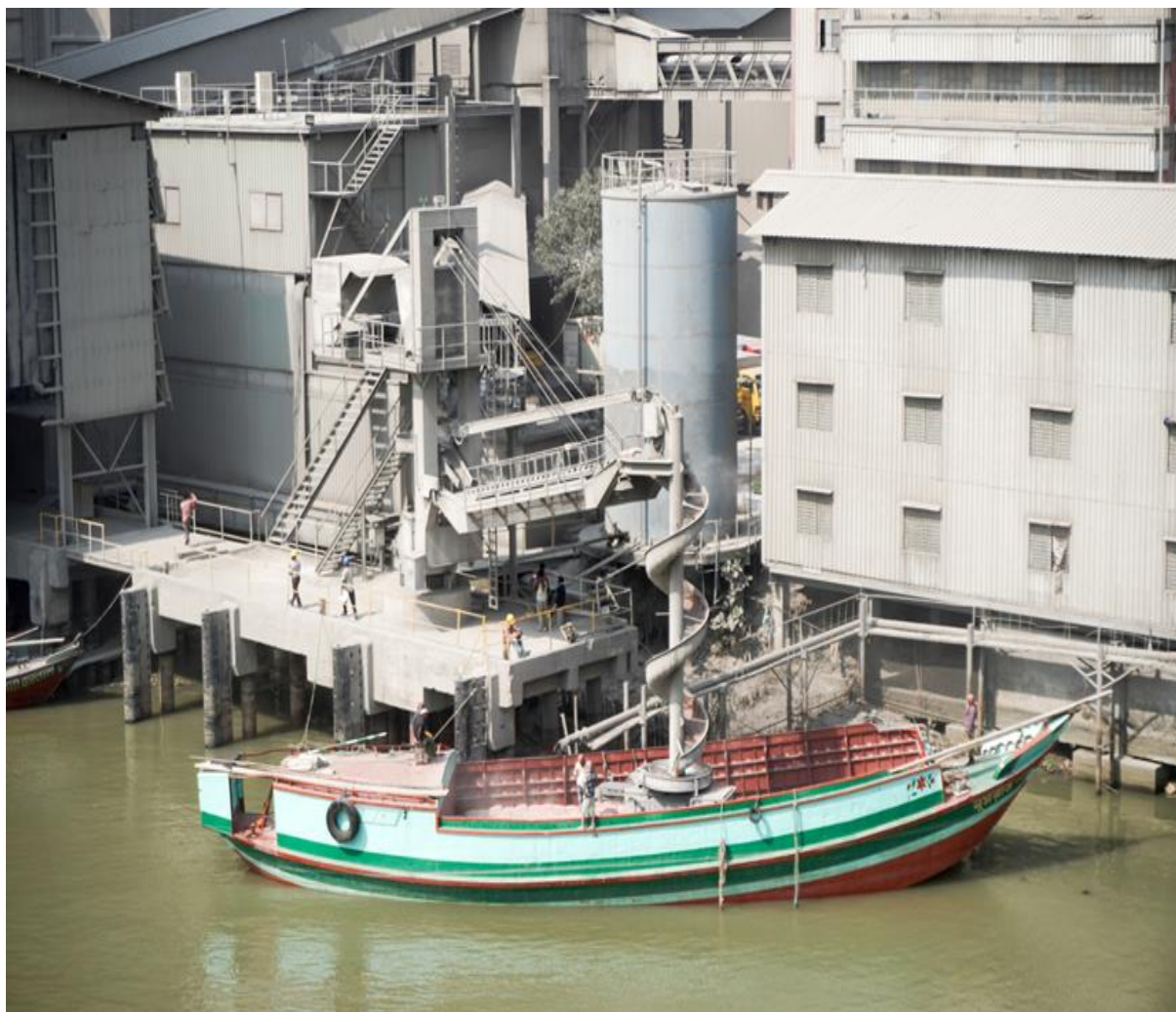
Figure 2: This picture shows the distribution of produced cement directly from the factory to the distribution vessel (a local boat). The laborers involved in this process took no precautions or protective measures. During this process there are common occurrences of leakage of cement and fly ash from the discharge hanger, Kanchpur, Dhaka. Source: ESDO, 2022.
