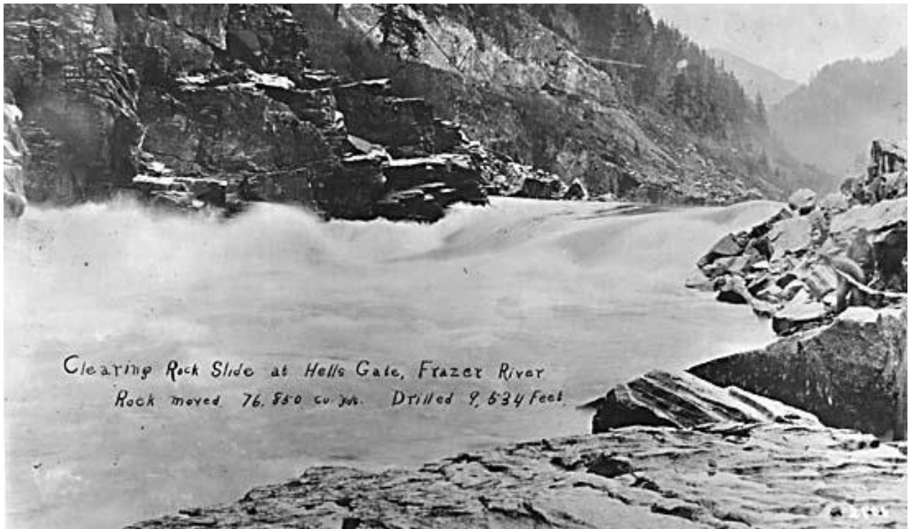
Figure 17: Clearing rock slide at Hells Gate, Fraser River circa 1910-1920 Source: Major Matthew Collection, Vancouver City Archives A-8-3.2
