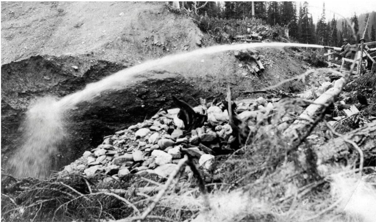
Figure 5: Hydraulic mining Source: Quesnel & District Museum http://www.quesnel Exhibits.ca/images/mining/picture4.jpg
