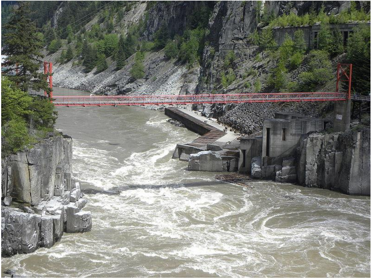
Figure 18: Fraser River Hells Gate, with constructed fish ladder visible on righthand side of river. Source: https://commons.wikimedia.org/wiki/File:Hells_Gate.jpg D Harvey Creative Common Attribution-Share Alike 3.0 Unported license
