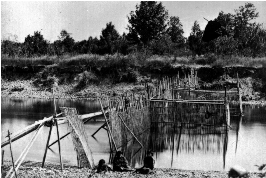
Figure 3: Typical type of First Nations salmon weir. Source: Image G-06604 Royal Museum, BC Archives
