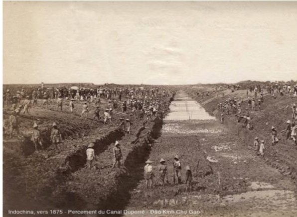
Figure 7: The excavation of Cho Gao Canal in 1875. Source: www.anhxua.vn
