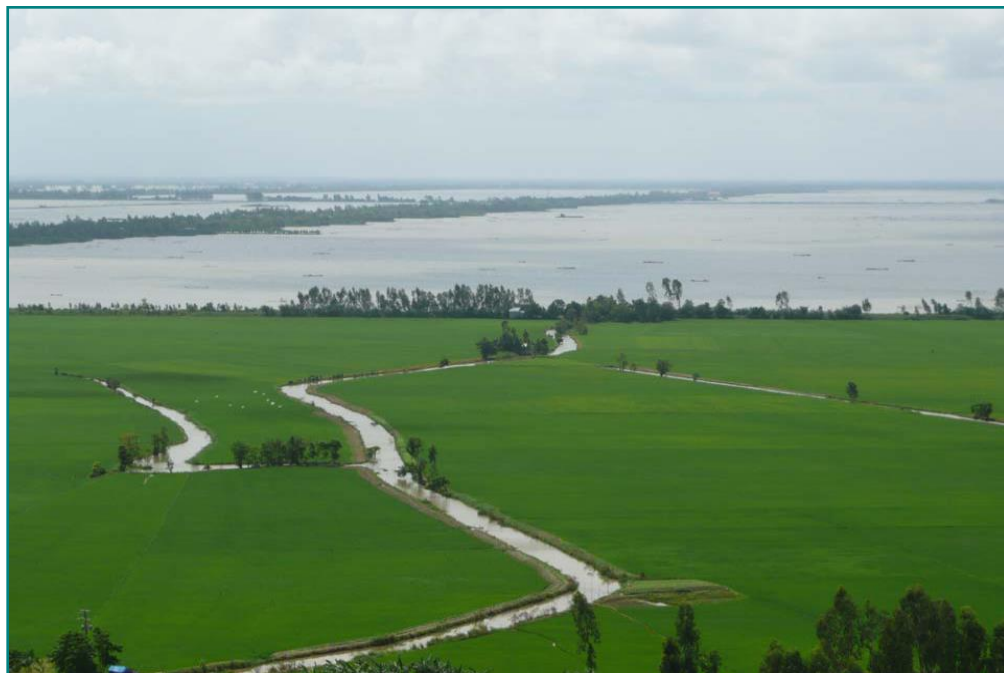
Figure 13: High dyke systems for additional rice production during flood season in An Giang province. Source: Tran Xuan Long
