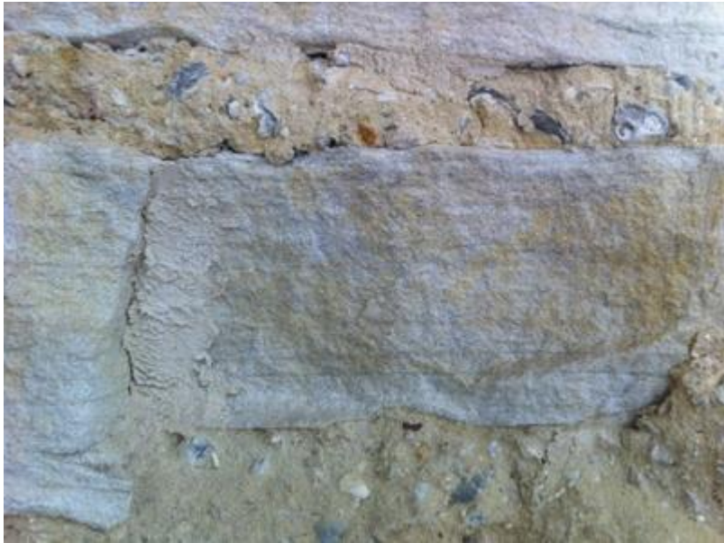
Figure 4: Oyster shells in the mortar in the Laundry Vacluse House built around 1820s © Sydney Living Museums / Historic Houses Trust
