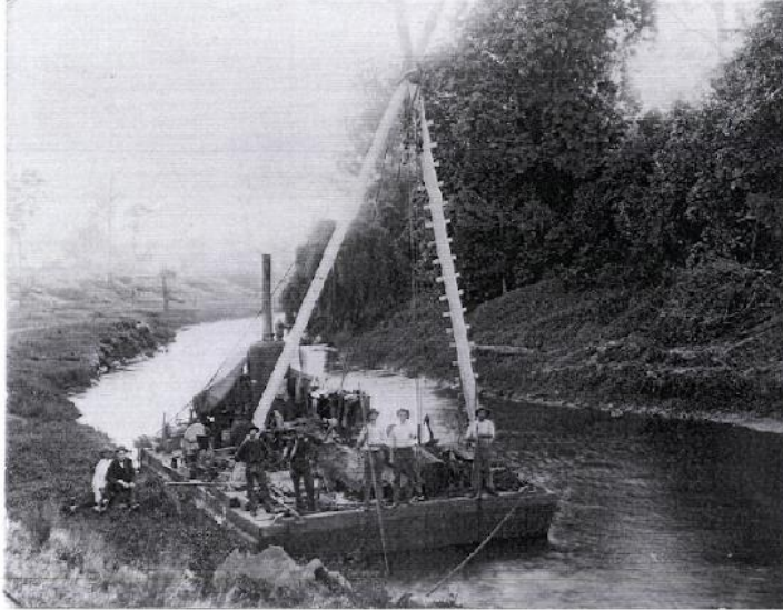
Figure 7: Upper Richmond River de-snagging barge circa late 1800's. Note the complete loss of riparian vegetation and in-stream timber habitat. Source: Richmond River Historical Society
