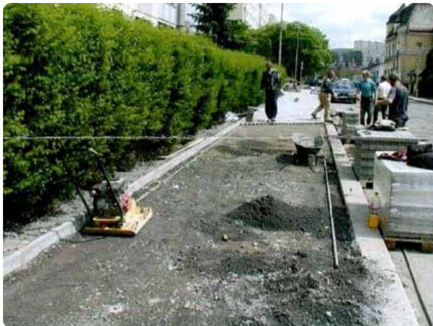
Figure 26: Promotion of use of mixed fly ash and bottom ash as a foundation for sidewalks in the Czech Republic. Levels of PCDD/Fs in this mixture are about 0.05 - 0.1 ppb in WHO-TEQ. Source: Letter sent by company Termizo, operating MWI in Liberec to mayors in the region.
