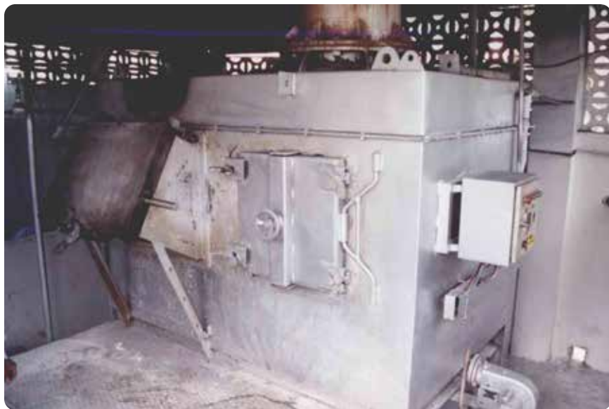
Figure 39: Double chamber furnace in one of small MedWI in Pakistan. Photo by Jindrich Petrlík, Arnika, March 2005.
