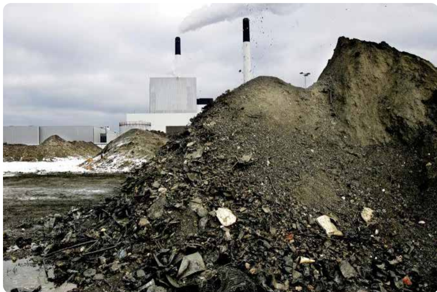
Figure 1: Waste incinerator in Copenhagen with pile of bottom ash; In many EU countries is bottom ash used for roads construction and pavement. In some cases it also includes fly ash. Source: (Borking 2011).
